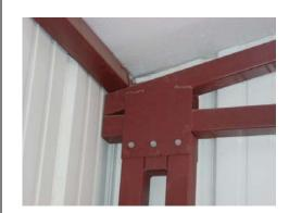
Leg assembly for side wall and O.H. Door
